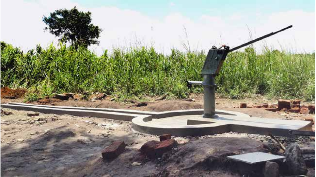
Borehole repair, almost complete
