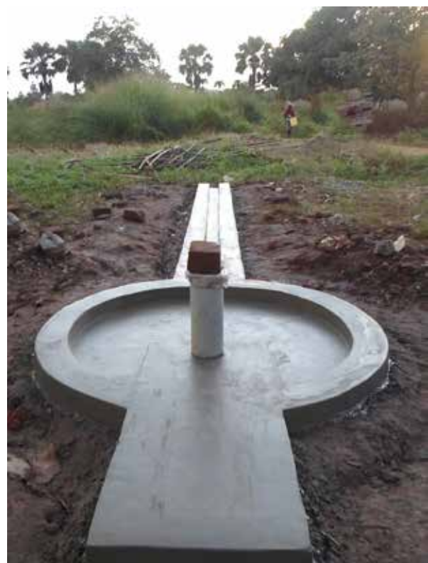
Freshly poured borehole foundation.
