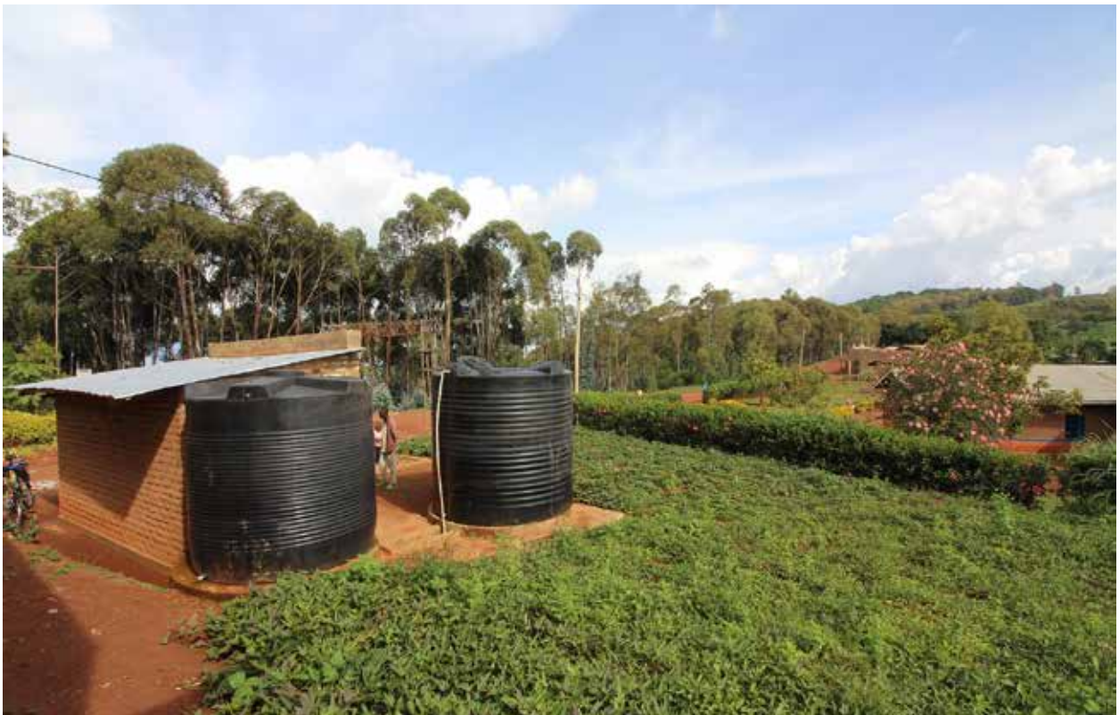
Water storage tanks.
