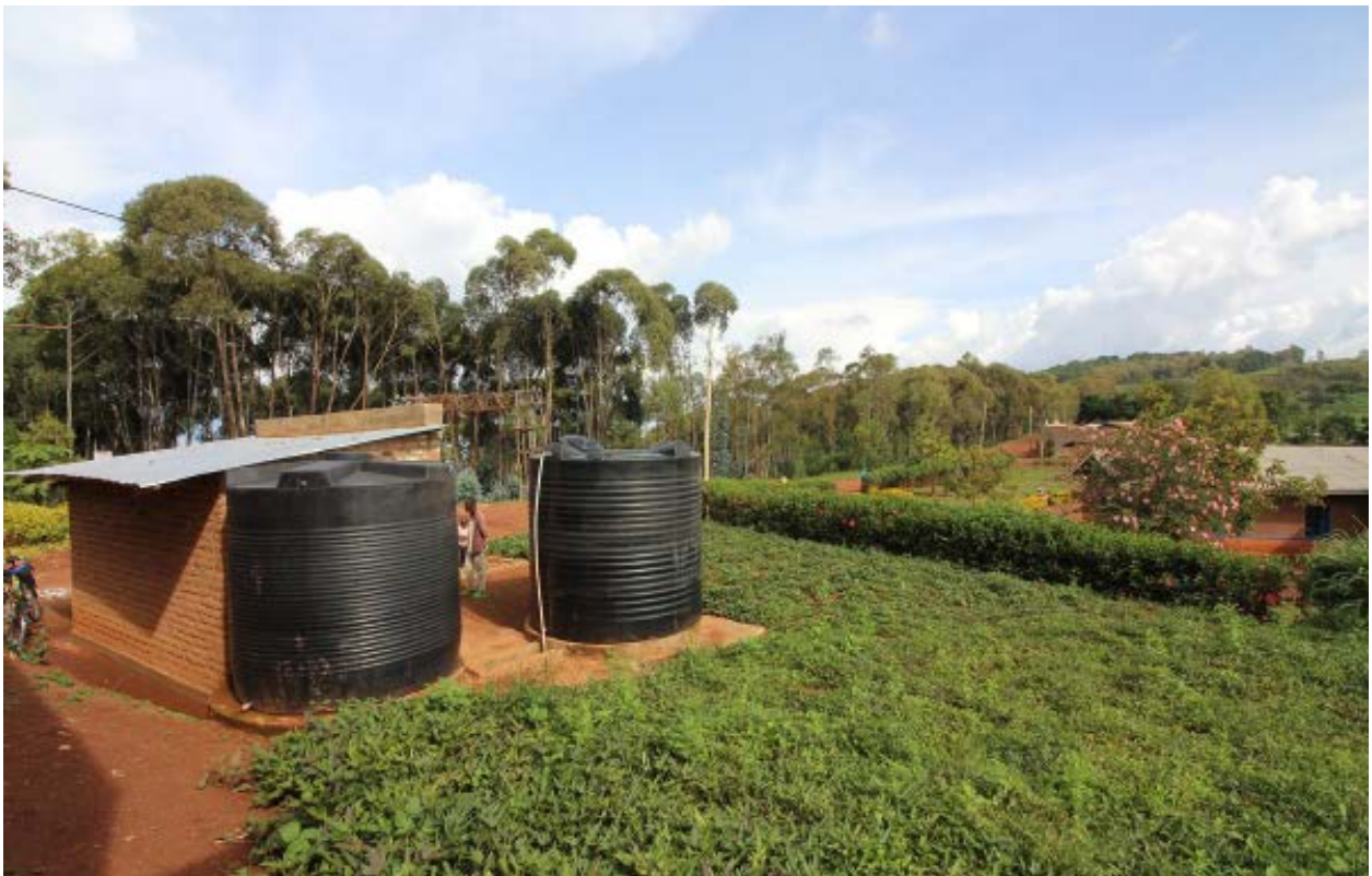
Water storage tanks.
